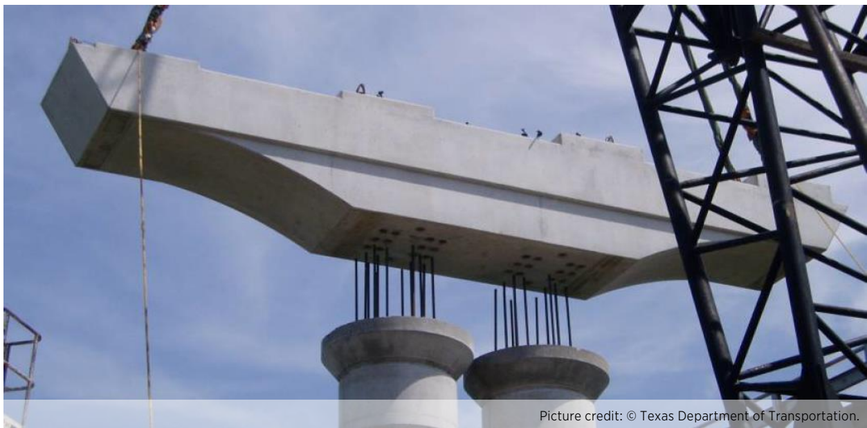
Figure 22 Connection between Columns and Cap Beam
