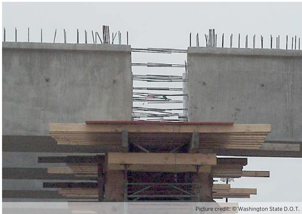
Figure 16 Transverse Connection between Beams in Field
