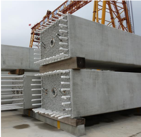
Figure 30 prefabricated element reinforcement part, connection prior to connection
