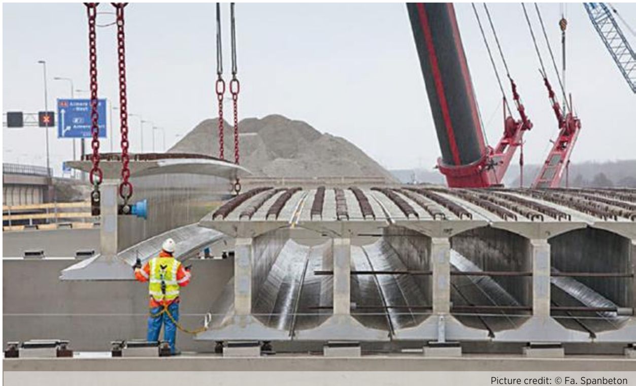
Figure 11 Adjacent Butted Tee Beams
