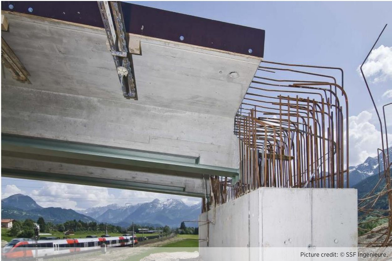
Figure 19 Integral Connection between Superstructure and Abutment
