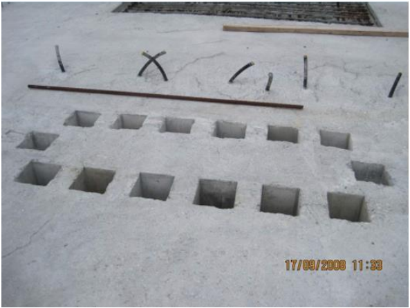
Figure 21 Connection between Column and Bridge Deck [U8]
