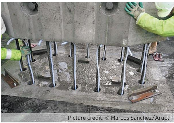
Figure 34 Connection of Column to Footing
