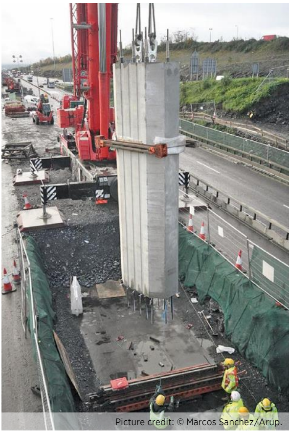
Figure 33 Connection of Column to Footing
