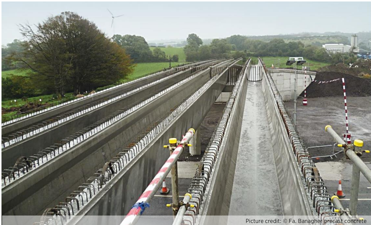
Figure 10 U-shaped Beams in a Decked Stringer System
