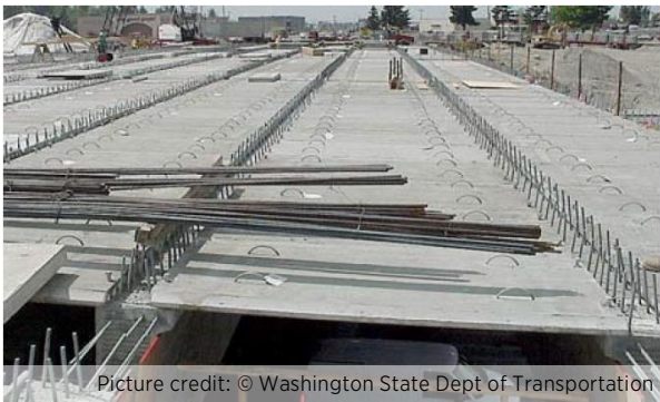
Figure 6 Partial-Depth Precast Concrete Deck Panels
